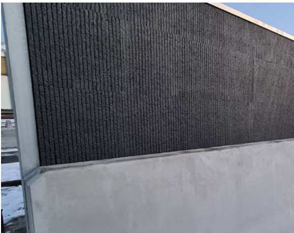
Application as facing shell e.g. for renovation of existing noise barriers
